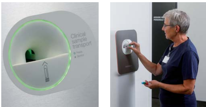
Sample tubes are placed in the insertion point of the Vita.
